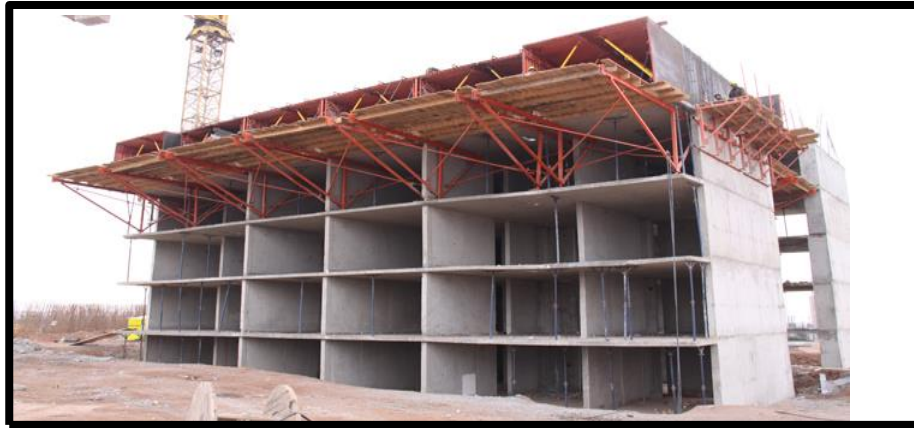
Figure – 95 Tunnel formwork system
