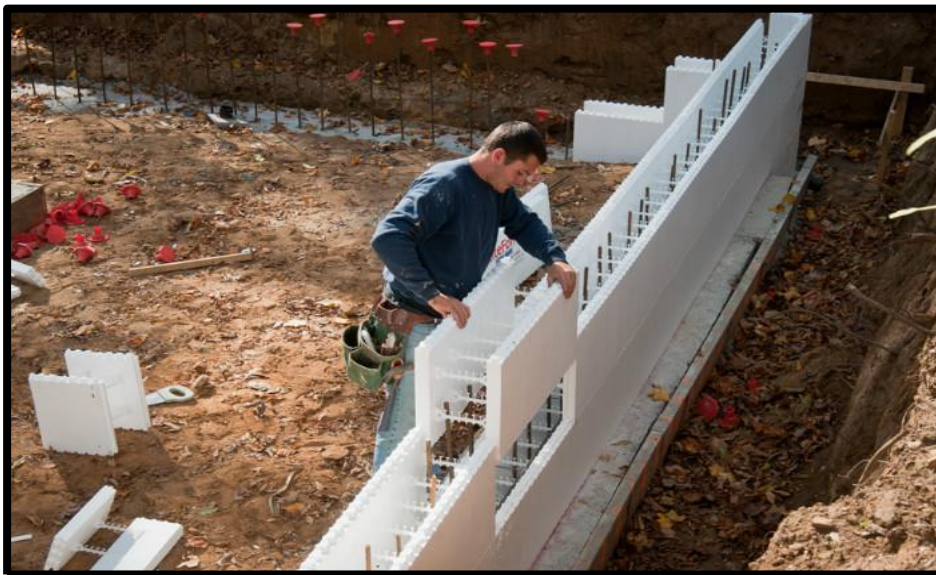
Figure - 98 Insulating concrete formwork technique
